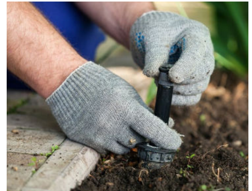
Check sprinklers and irrigation
